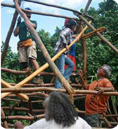
MNBG Horticulturalist Kaili Kosaka helps install ahū pueo (cross beams) with Palani Sinenci directing.
